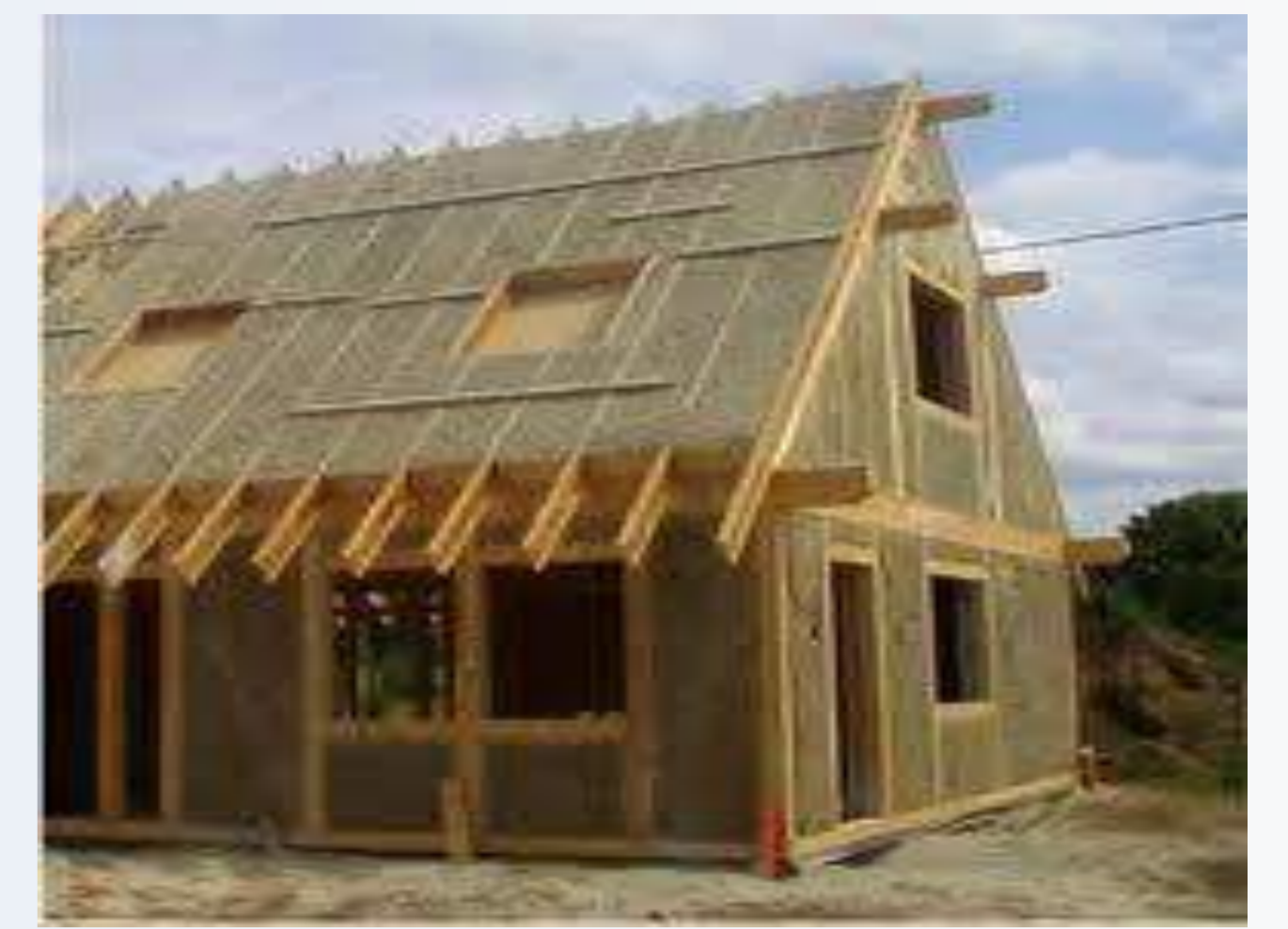
Hemp concrete as infill material in timber walls.
